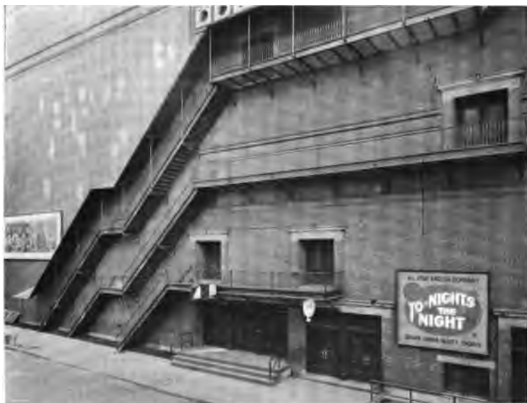
Fig. 3. Protected outside Stairways "Straight-Run" Type.*
